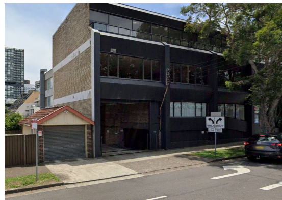
Existing garage entrance - proposed location unchanged
